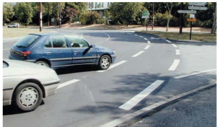
2-lane and 3-lane entries and exits on the circle = danger (FFCT J. Fourna)
