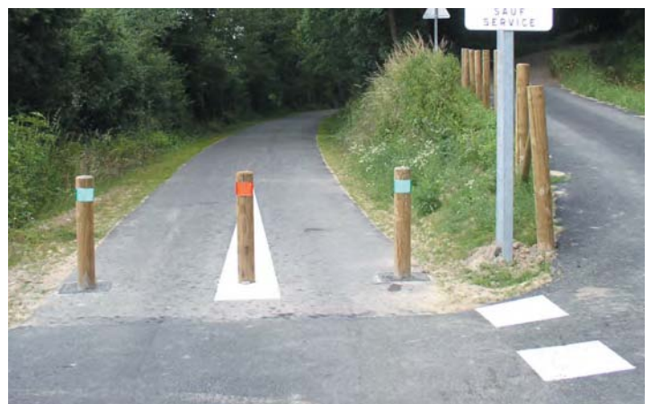
0.9-m bollard with reflective band (CG 69)
