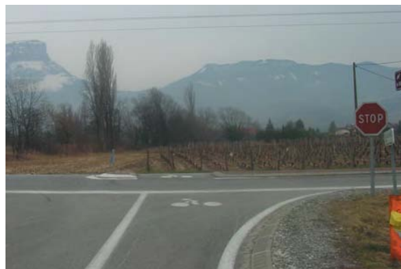
The lane is kept ; the T3 5u turns into a solid line (Cete Lyon)
