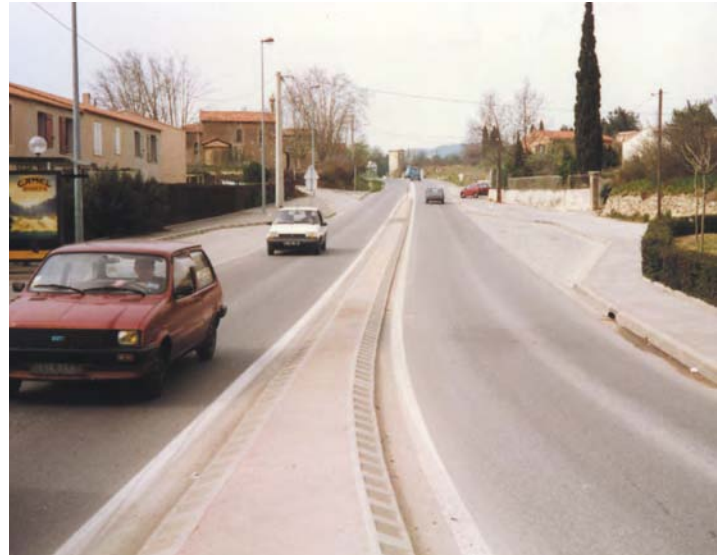
The island reinforces the straight-line effect to the detriment of cyclists (Cete Méditerranée)
