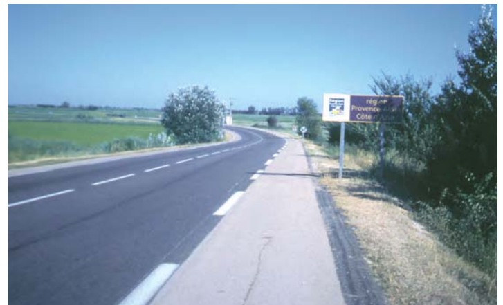
Colouring optically narrows the carriageway width (Certu)
