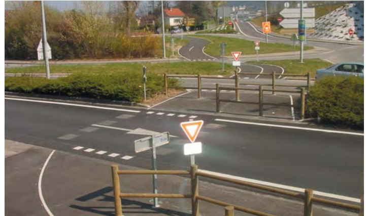
National trunk road redeveloped to make the greenway safe (Cete Lyon)
