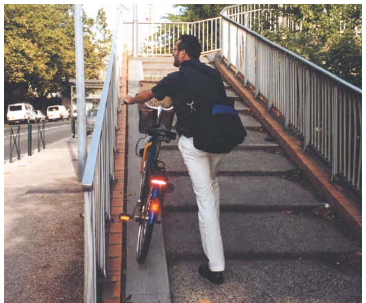
A small ramp enables bicycles to be pushed effortlessly along a staircase (Certu)
