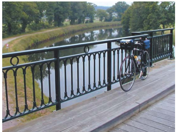
1-m barrier sufficient, however surface unsuitable for rollerblading (FFCT J. Fournat)
