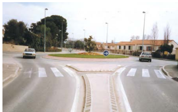
The natural position of the cyclist is in the centre of the circular roadway (Cete Méditerranée)
