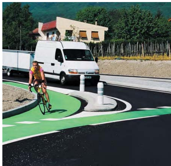
The cycling space is clearly identified and respected (optional green colour) (FFCT J. Fourna)
