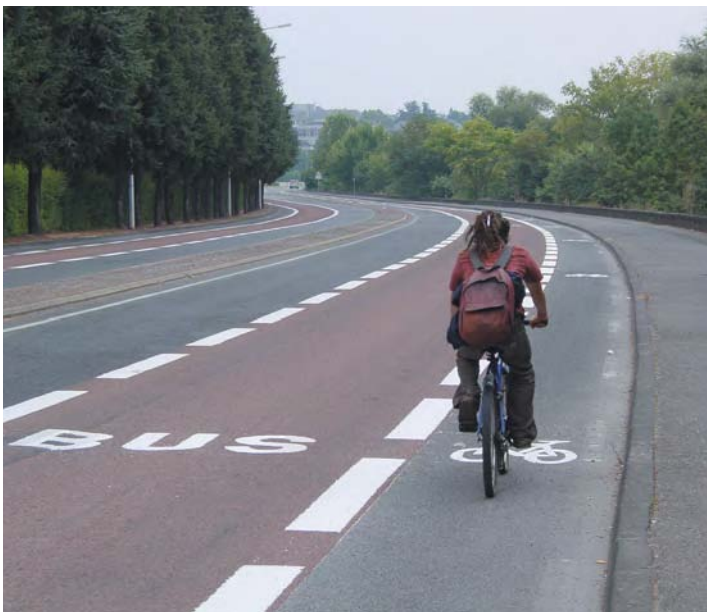
A form of road-sharing which is appropriate in periurban areas for well-spaced bus stops
