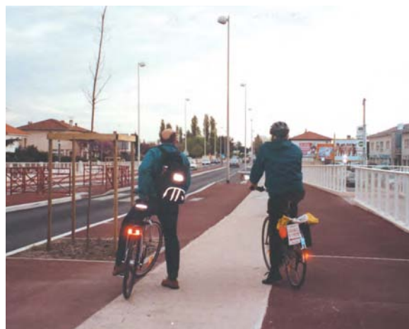
Few house frontages and wide pavements - a good opportunity for a pavement cycle path (Certu)
