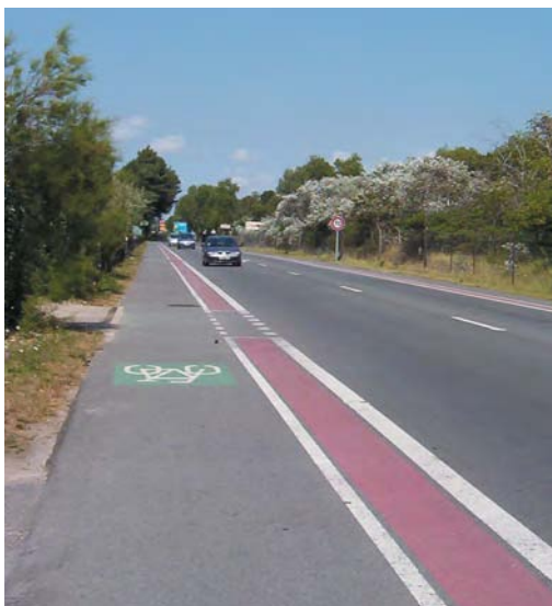
A lane that is almost as comfortable as a path (non-statutory marking) (Cete NPC)
