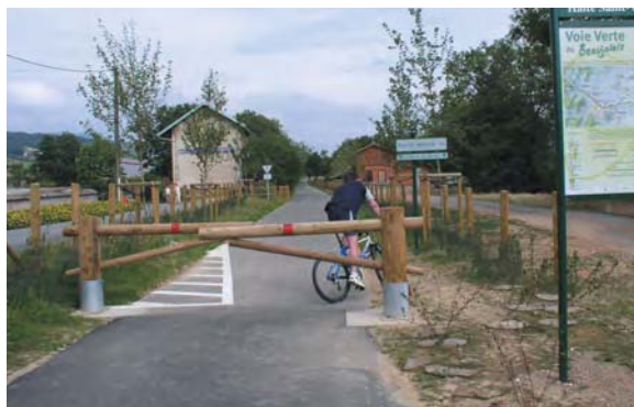
Backing up the horizontal and vertical signage (CG 69)
