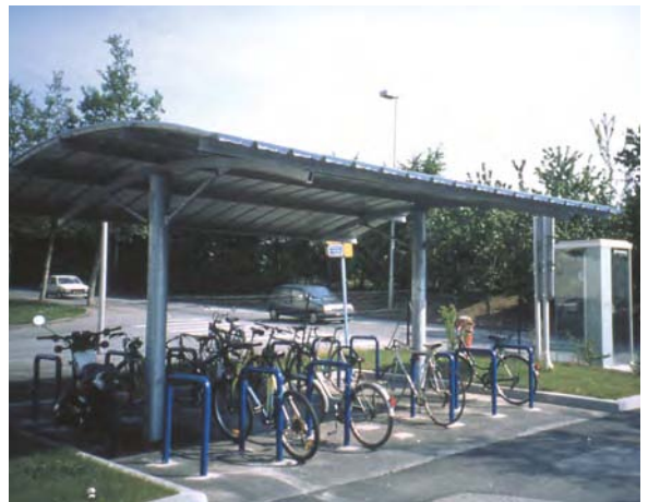
Sheffield stands are to be preferred over all other cycle hoop systems (ST Lorient)
