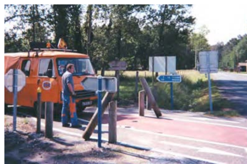
Maintenance operation on a greenway (Cete S.O.)
