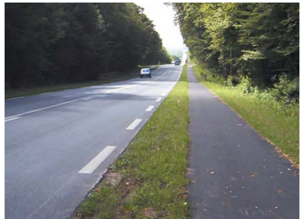
Quite suitable if there are few intersections and a regular cleaning programme (Cete NPC)
