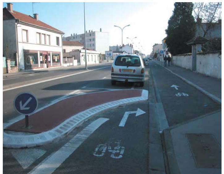
The deceleration island does not disturb cycle travel (ST Chalon-sur-Saône)
