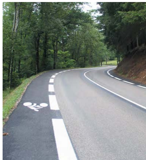
Hardstrips that easily convert into cycle lanes (CG 69)
