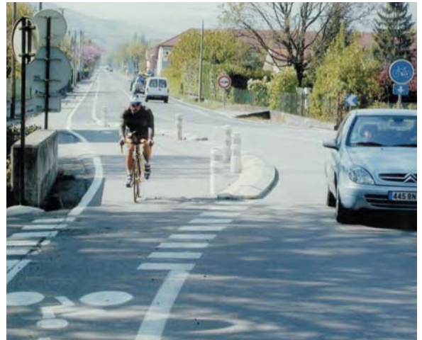
A chicane breaks the straight line of travel but islands ensure the space reserved for cyclists is seamless (FFCT J. Fourné)
