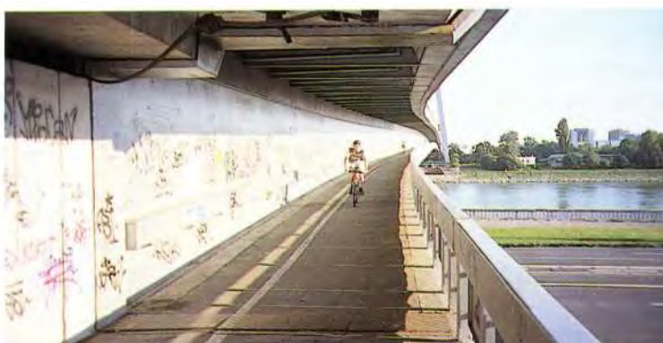
Cycle path on cantilever supports under engineering works
