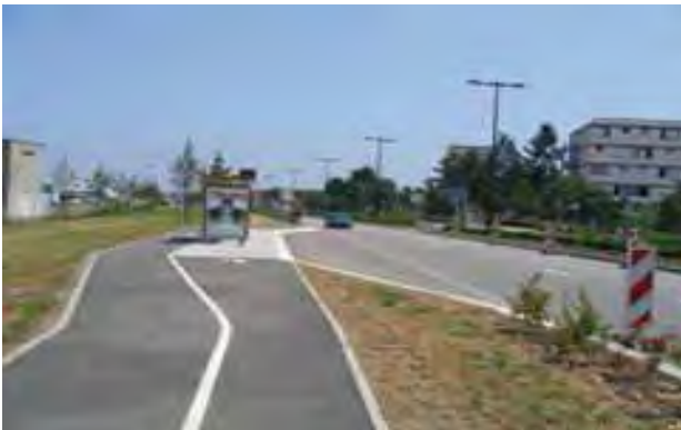
Lane behind a bus stop only if few pedestrians and little space
