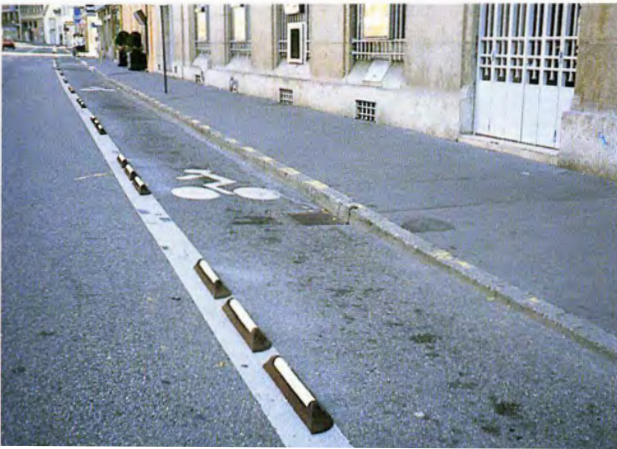
Rubber separator that can be crossed
