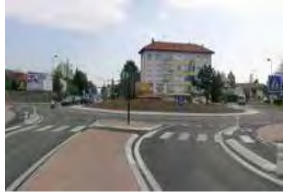
Handling a large roundabout with cycle lane
