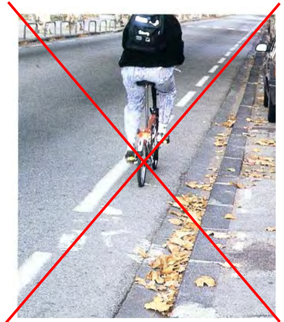
Cycle lane too narrow
