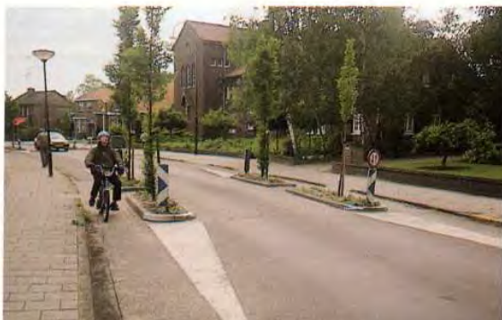
Pinch point with bypass
