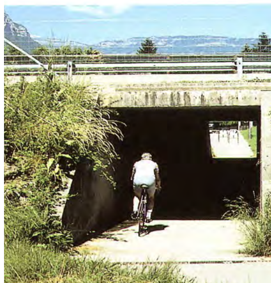
Continuous route with underpass
