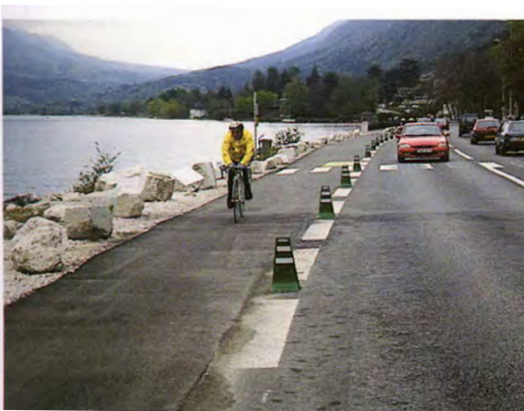
Flat posts alongside Annecy Lake
